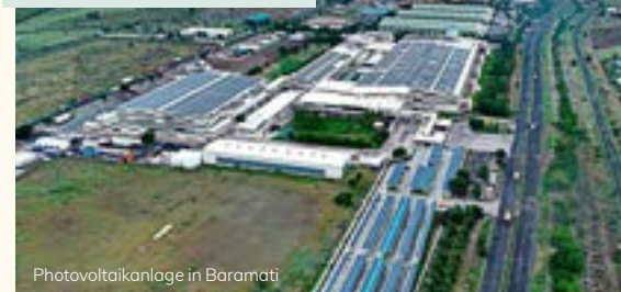
Photovoltaikanlage in Baramati
